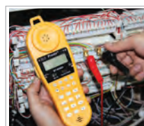
Telephone line testing
