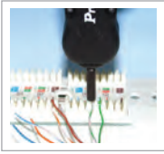
Punch and cut cable terminals
