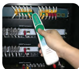
Copper cabling detecting
