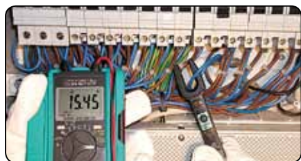
Measuring current in a Switchboard
